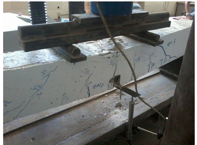
Figure 14. Crack Pattern for One of Tested RC Beams (as an Example)
